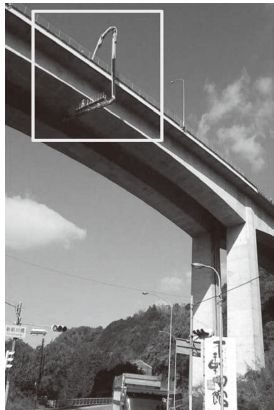
Photo 2 Example of bridge inspection.
